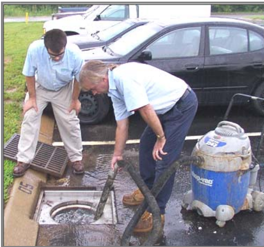
A shop vacuum is used to clean an Aqua-Guardian™ Catch Basin Insert
