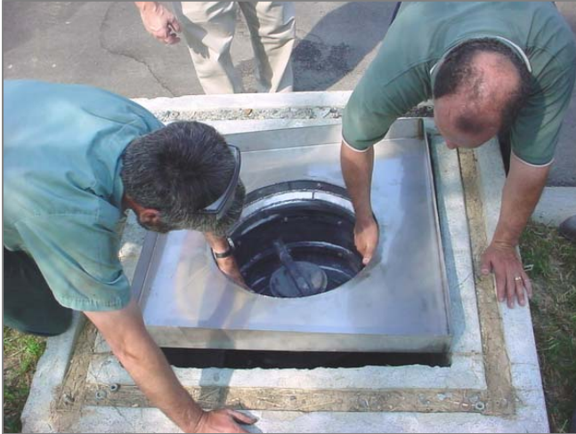
Simple installation of an Aqua-Guardian™ Catch Basin Insert
