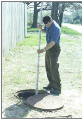
Sediment inspection using a stadia rod
