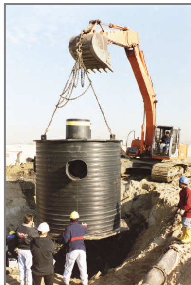
The Aqua-Swirl™ installed using a trackhoe
