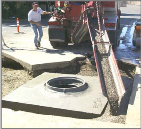
Concrete pad protects the Aqua-Swirl™ from impact loading
