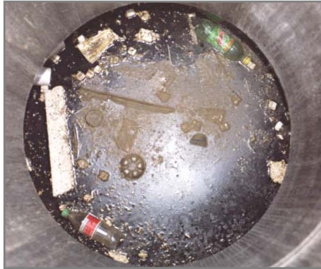
Floatable debris in the Aqua-Swirl™
