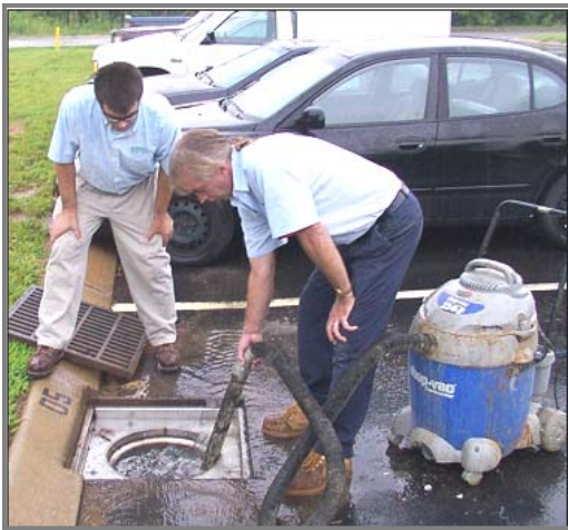
A shop vacuum cleans an Aqua-Guardian™ Catch Basin Insert
