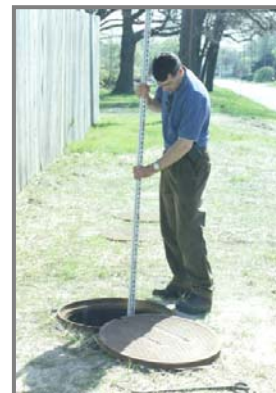
Sediment inspection using a stadia rod
