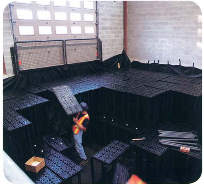
StormTank installation used for structural load testing.
