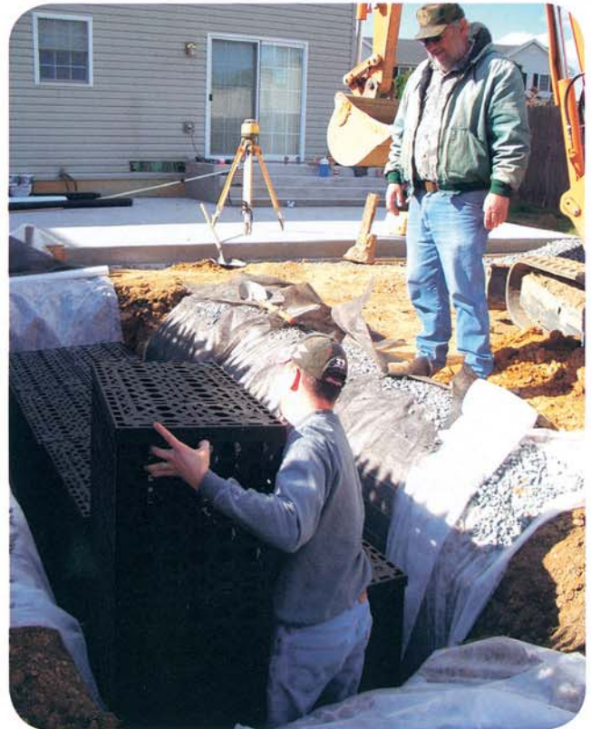
Residential installation of plastic modules for onsite infiltration.
